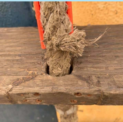
Worn and frayed side rope at pilot step.
